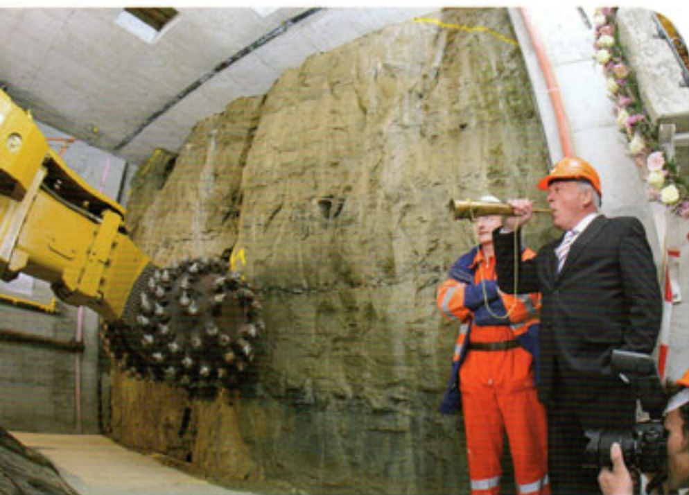
Fritz Wyss, then Head of Administration at Emmi AG, gives the signal for the construction work to begin.
